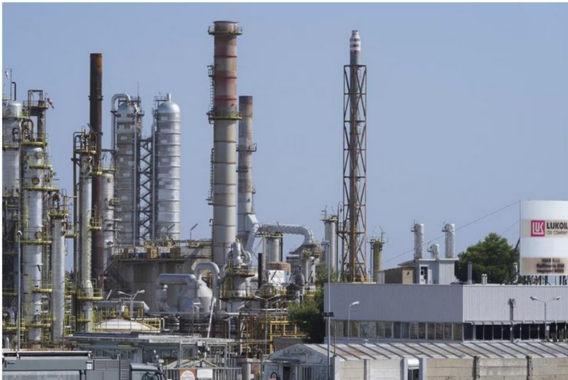
General view of the ISAB plant, the Lukoil-owned oil refinery in Sicily, Italy October 27, 2022.
