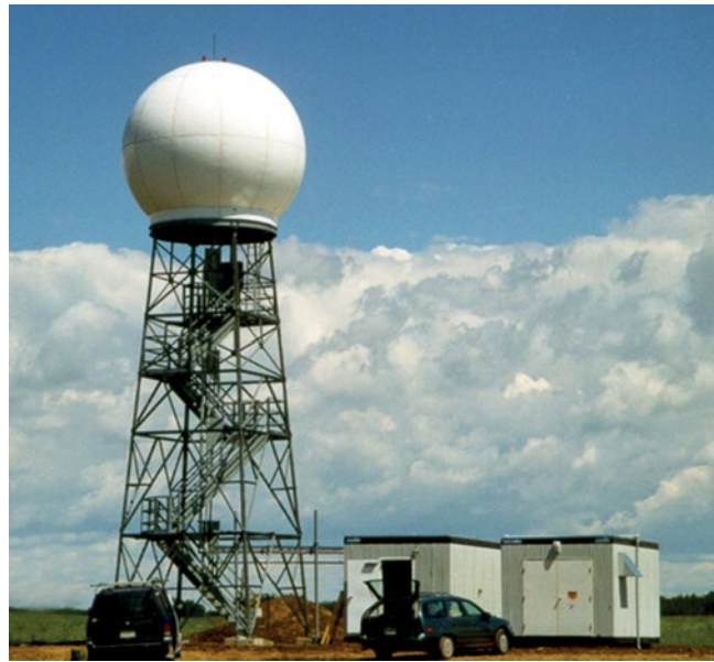
Figure 7.1. A typical weather radar within the Canadian network showing the major physical components of a radar system. The tower is about 30 m high, with a radome fitted with hazard lights and a lightning rod.
