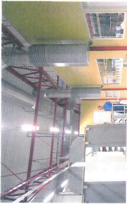
FIGURE 45. Displacement diffusers with both horizontally and vertically oriented spread patterns.
