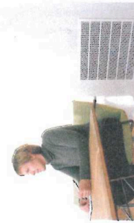
FIGURE 43. A diffuser built into a wall.
