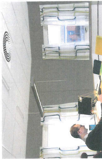
FIGURE 20. A ceiling mounted supply ATD in an office environment.
