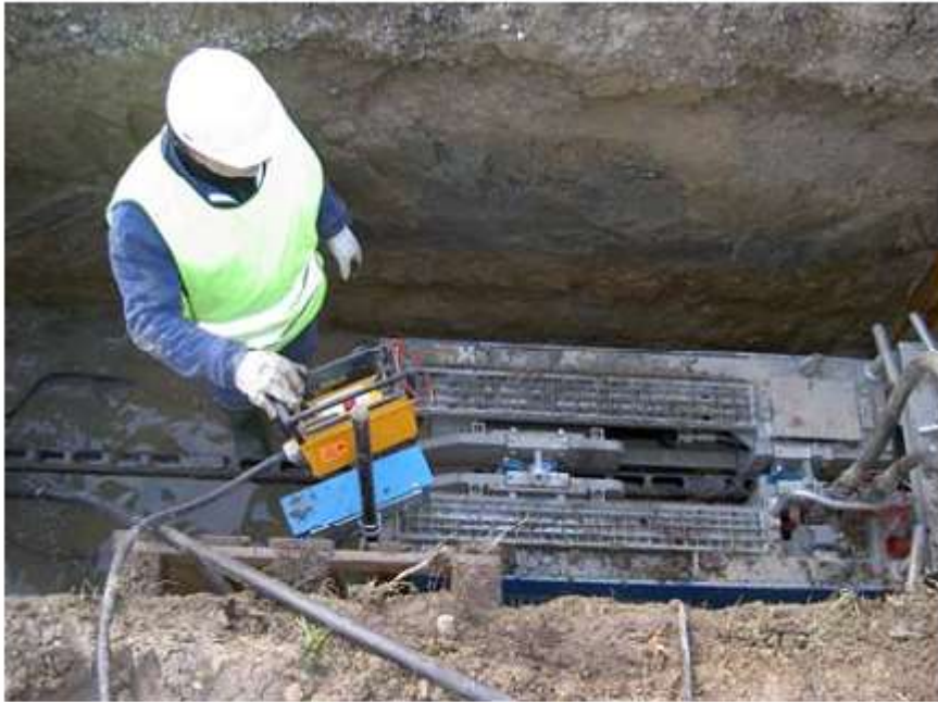
equipment used for pipe bursting work via Plebscito and in the Sheraton area in Padua
