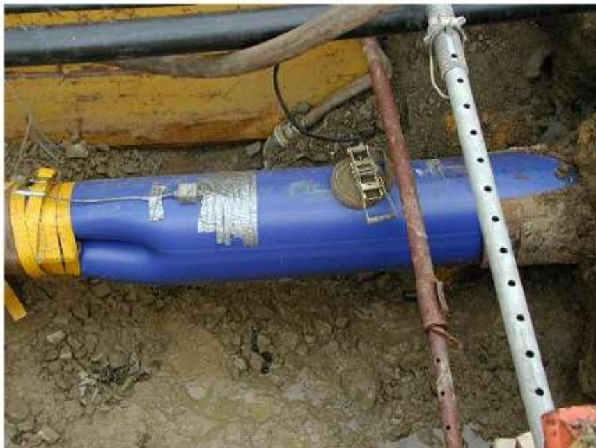
Insertion, steaming and final connection of an old water pipe with application of C-Compact PEHD pipe
