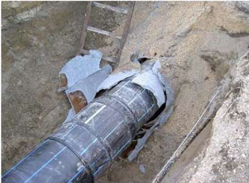
sequence of stages in pipe bursting
