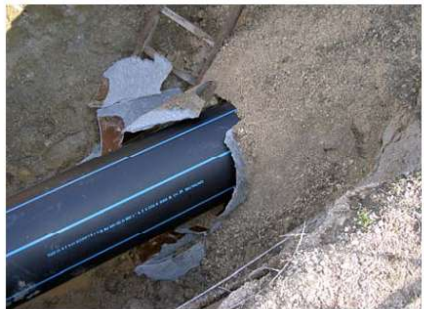
sequence of stages in pipe bursting
