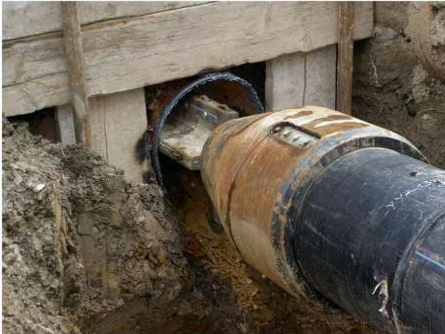
stages in application of pipe splitting for replacement of an old culvert under a road
