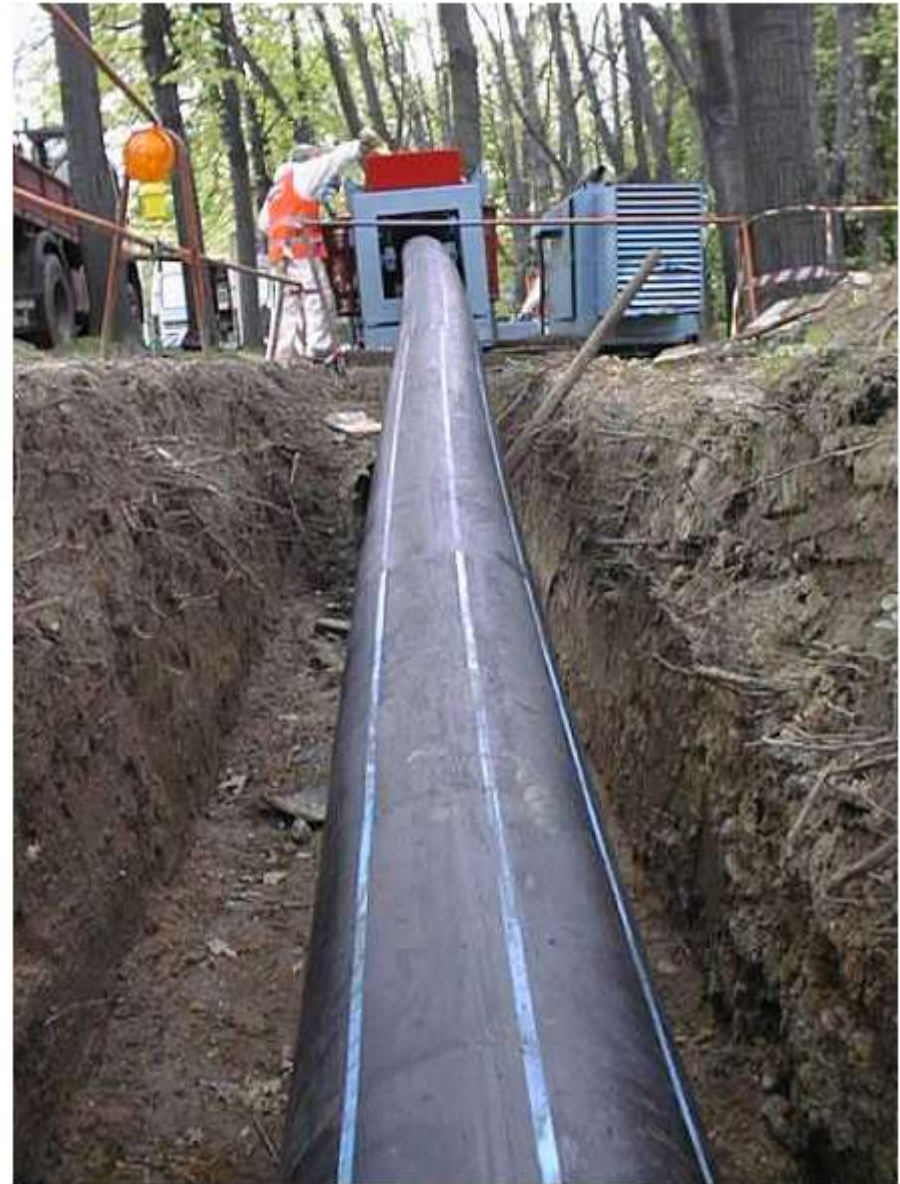
opposed rollers for reducing diameter and insertion of drawn pipe
