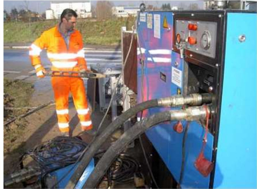
equipment used for pipe bursting work via Plebscito and in the Sheraton area in Padua
