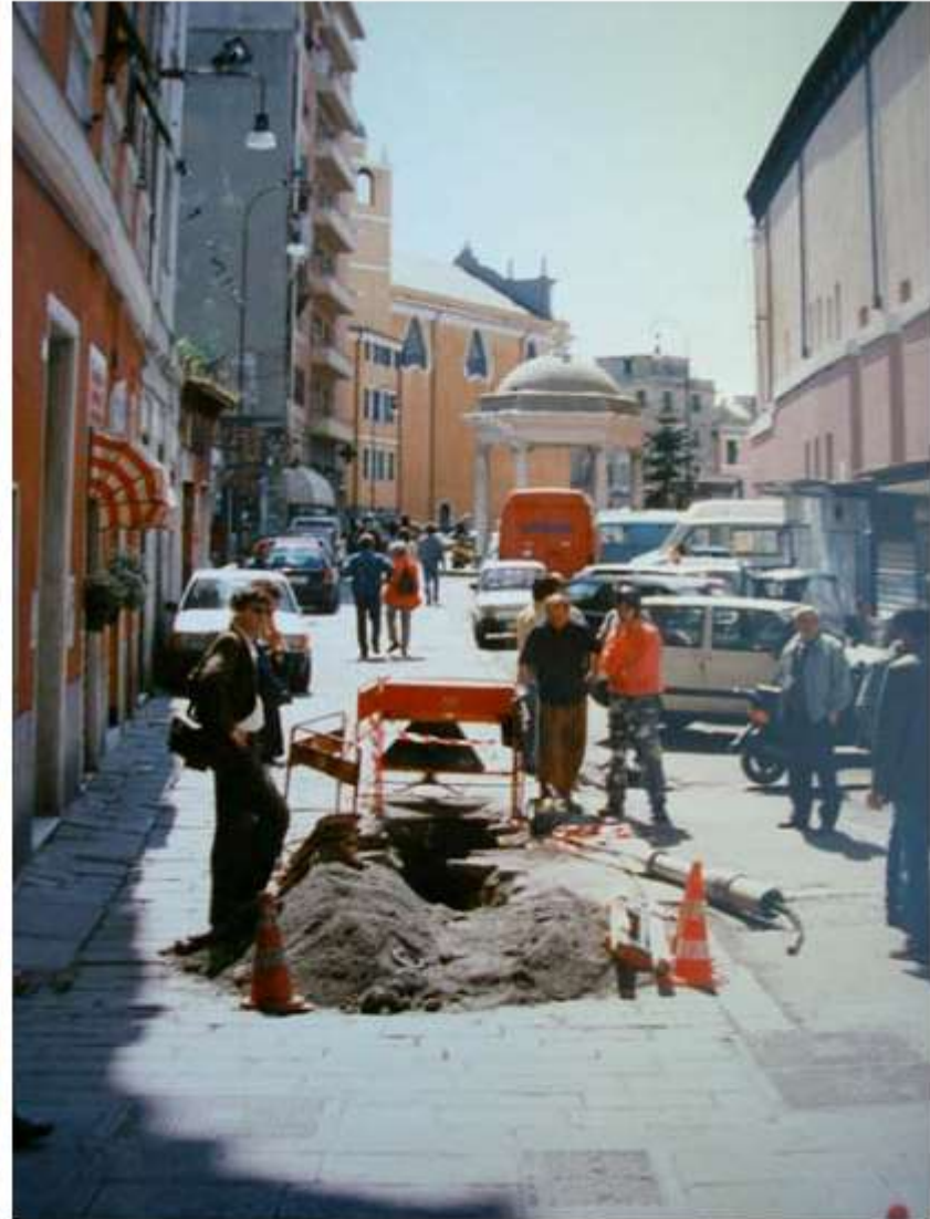
two archive photos illustrating the first No-Dig work in Genoa. Swage Lining DE500 mm in 1994 in the Circonvallazione a Mare area and the first experiment with Pipe Bursting in the old city centre, near S.Agostino theatre
