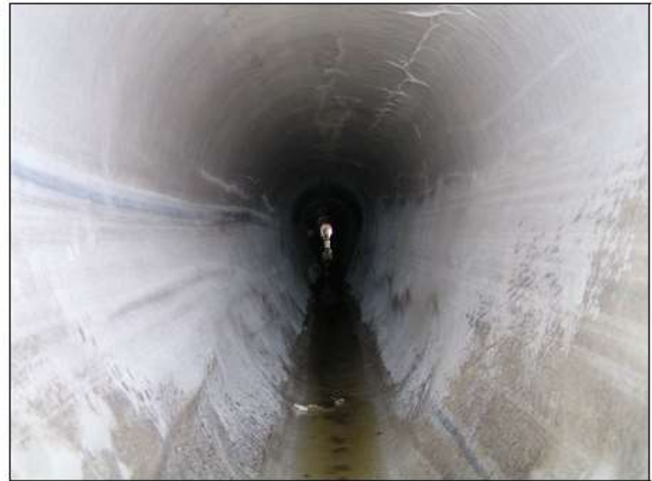
inside view of an oval-shaped sewer pipe before and after relining
