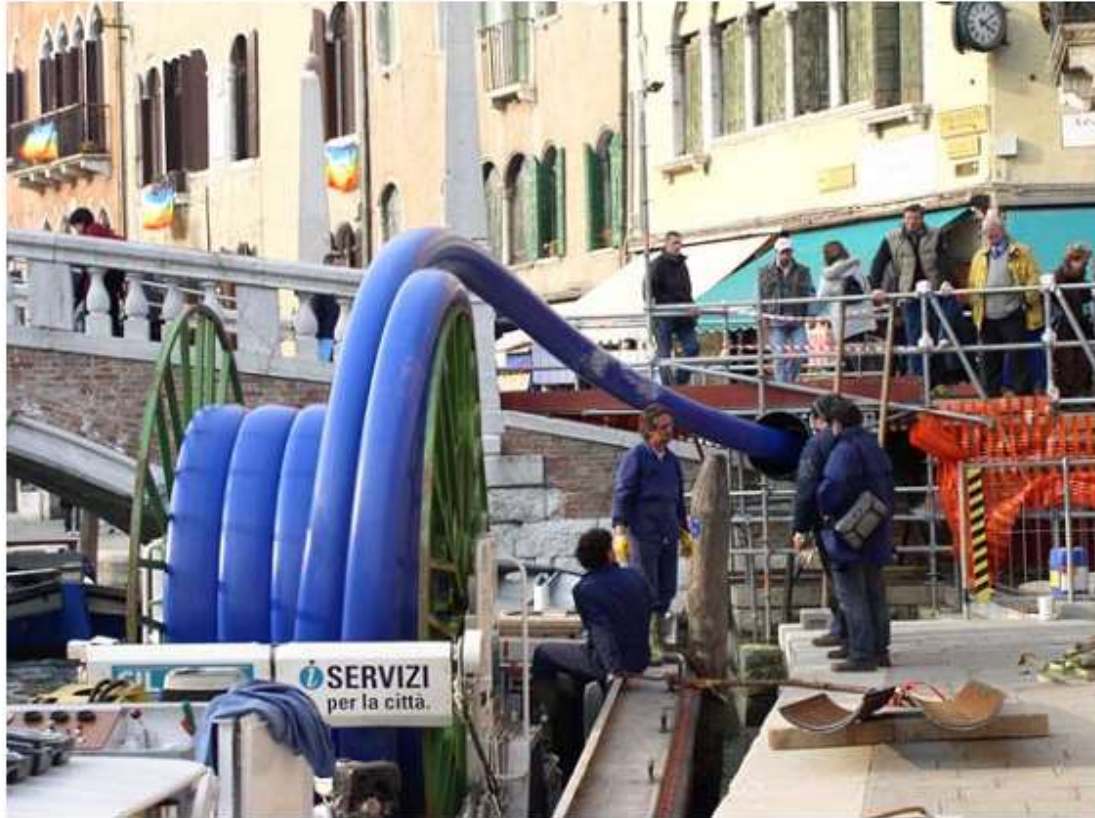
the C-Compact pipe is inserted in the pipeline, which runs perpendicular to the boat. A pipe with a wide curve is then prepared to aid its insertion
