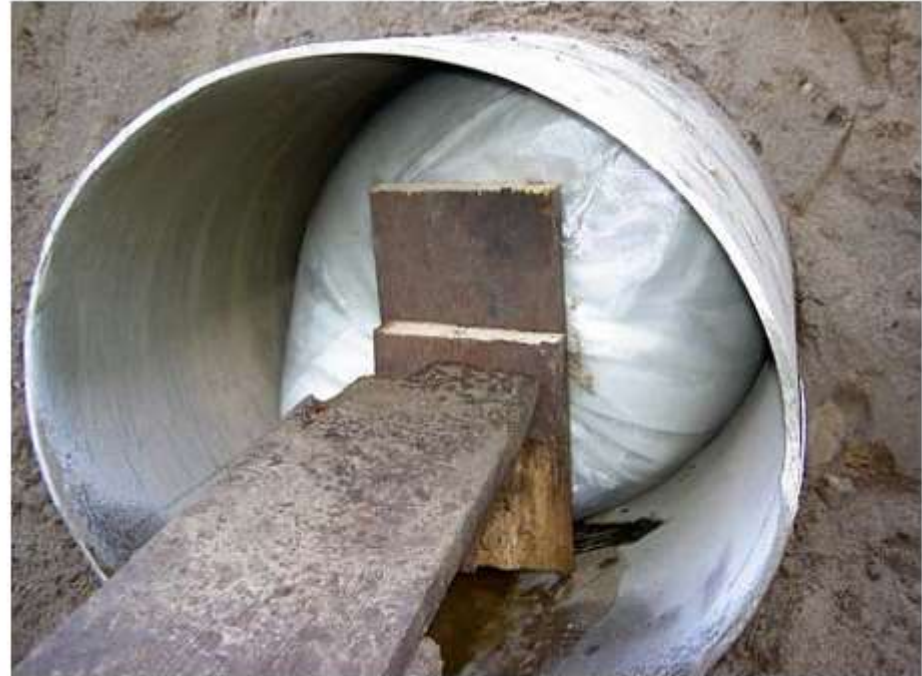
stages in application of C.I.P.P. thermosetting tubes
