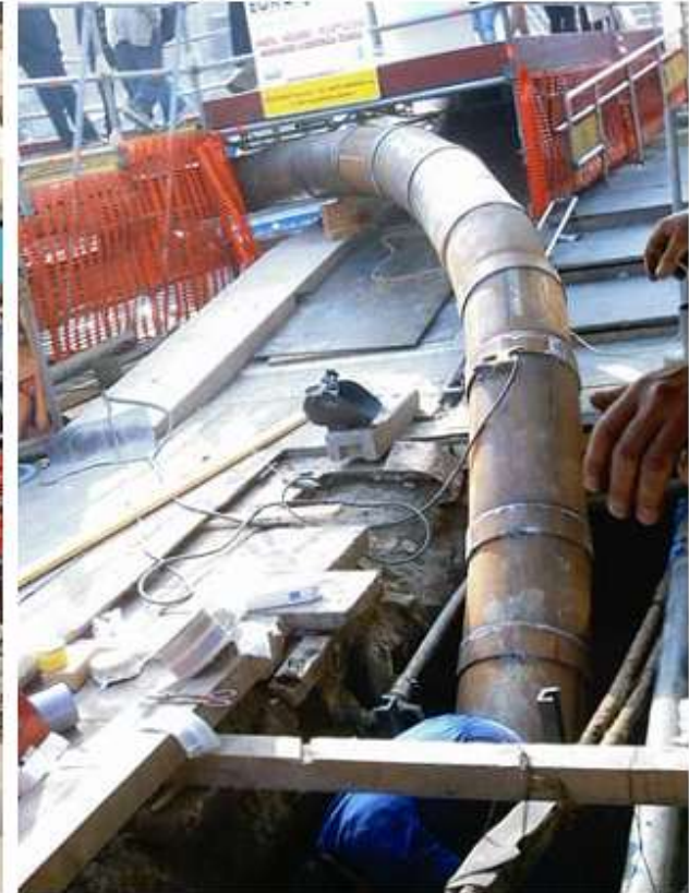
the C-Compact pipe is inserted in the pipeline, which runs perpendicular to the boat. A pipe with a wide curve is then prepared to aid its insertion
