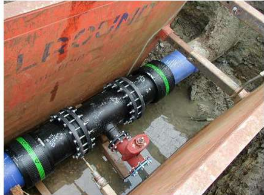
Insertion, steaming and final connection of an old water pipe with application of C-Compact PEHD pipe
