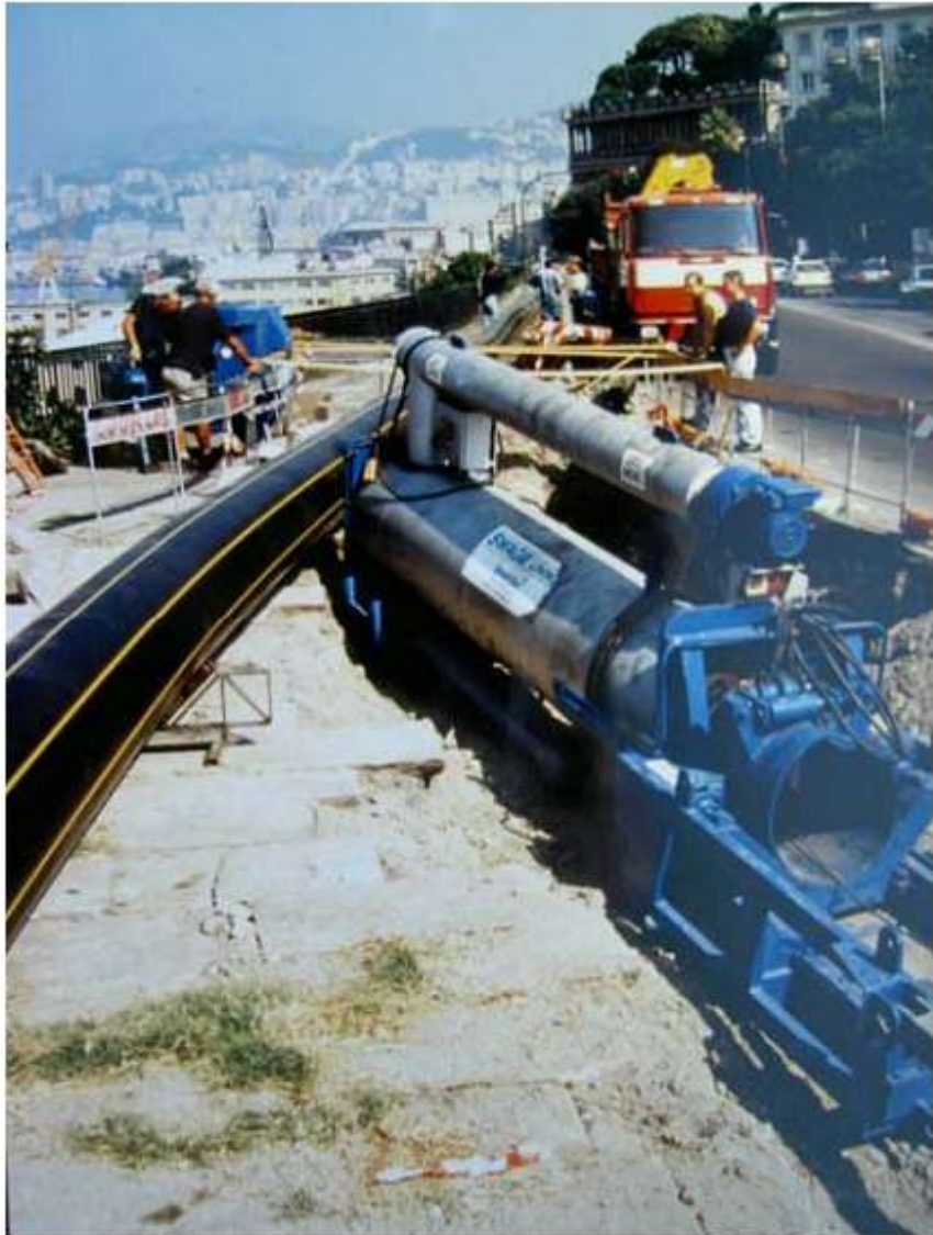
two archive photos illustrating the first No-Dig work in Genoa. Swage Lining DE500 mm in 1994 in the Circonvallazione a Mare area and the first experiment with Pipe Bursting in the old city centre, near S.Agostino theatre
