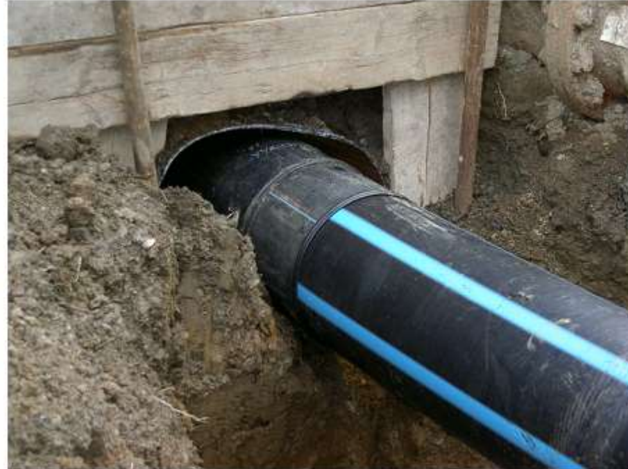
stages in application of pipe splitting for replacement of an old culvert under a road
