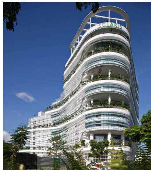
Fig. 10. An extensive 'green ramp' wraps around the building's façade (T. R. Hamzah & Yeang Sdn. Bhd.).
