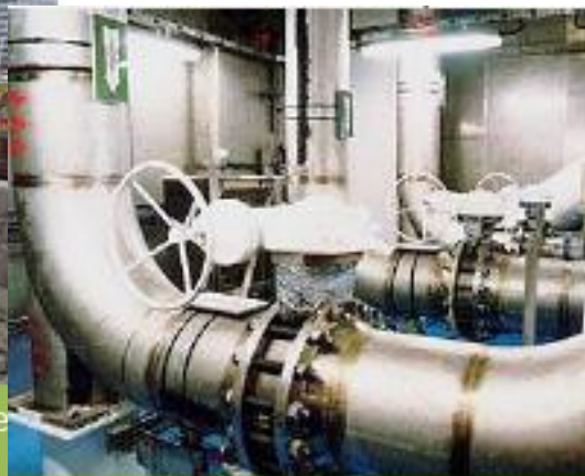
2507 used in Offshore seawater piping systems. Thanks to high strength and chloride resistance.
