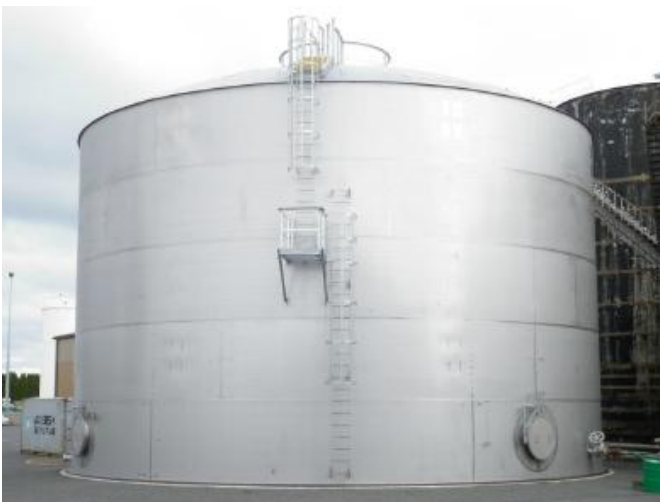
2101 used in Storage tank for a variety of media. Mechanical strength and good resistance in general being the reason for selection
