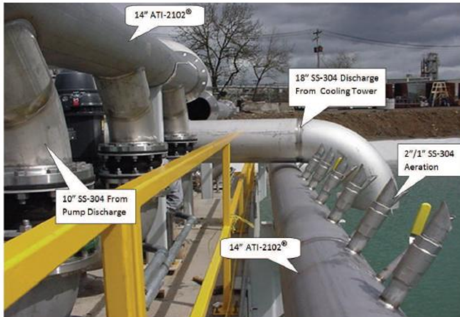
Figure 7: Detail showing locations of ATI 2102 ® LDSS and Type 304L.
