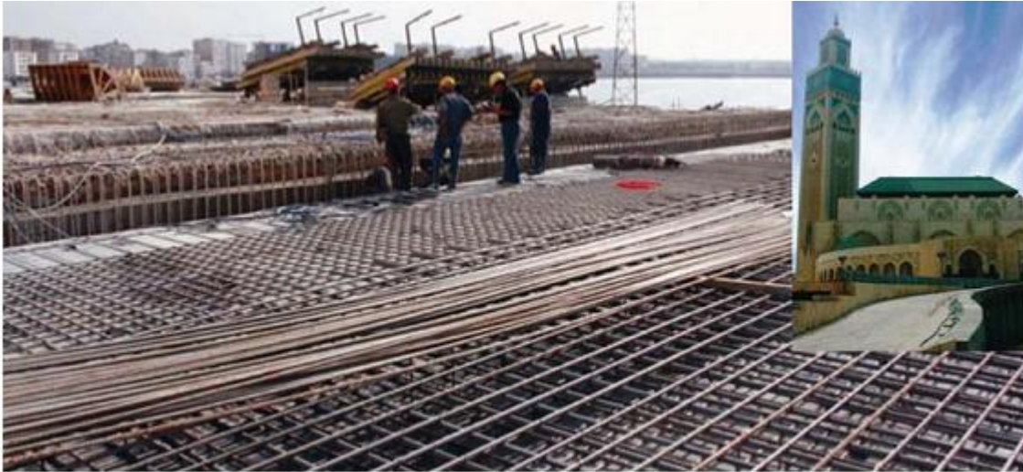
Figure 12. The great Casablanca mosque; more than 1500 tons of DSS rebar (2205 DSS).
