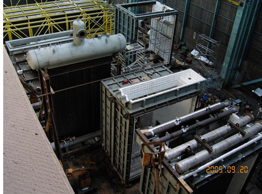
WHRS module assembly at site
