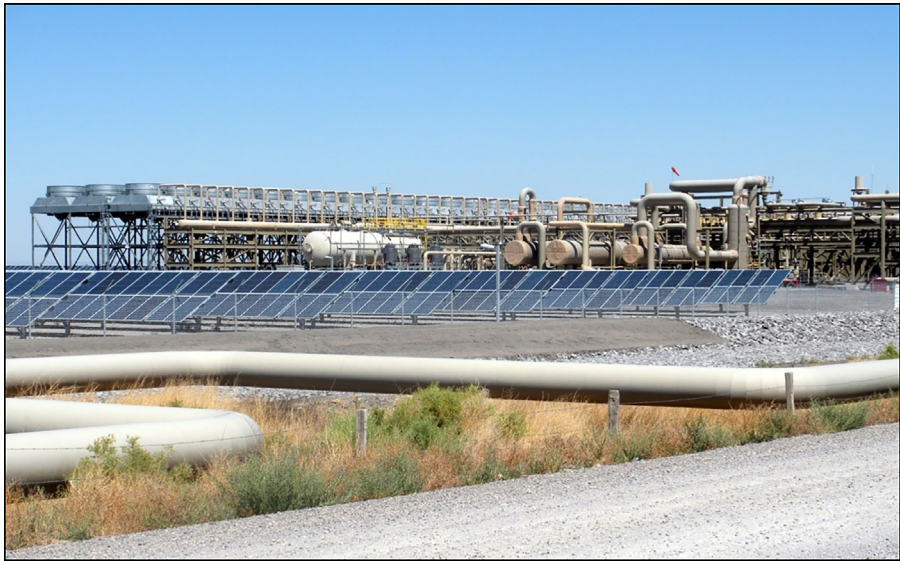
Figure 14.24 View of Stillwater binary plant showing a few of the 89,000 polycrystalline panels in the original PV system.
