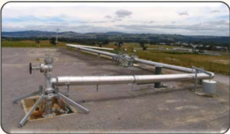
Production/ Injection Well
