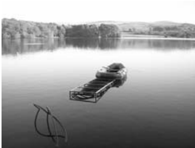
Figure 12.7 Coils for installation in a natural lake can be mounted in a steel frame, rowed out into the lake, filled and submerged. Photo reproduced by kind permission of Geowarmth Heat Pumps Ltd.
