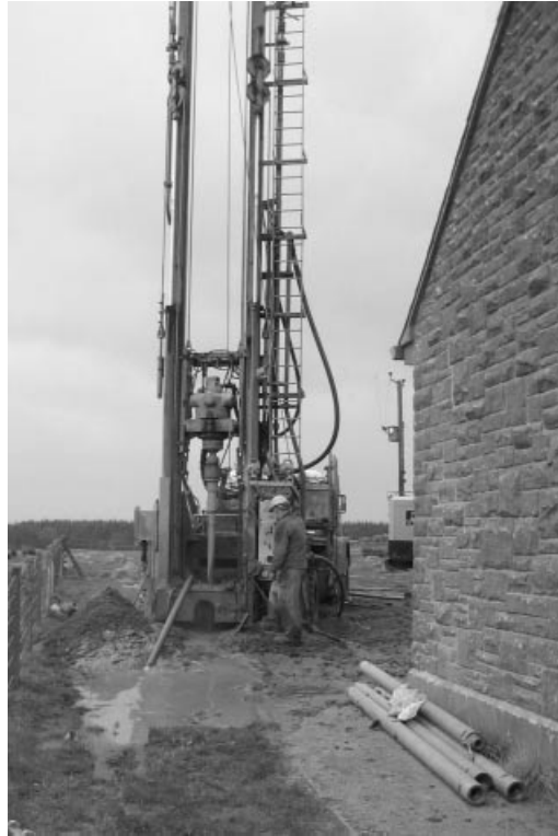
Figure 13.2 A down-the-hole (DTH) hammer rig in operation, drilling the standing column well at Grindon Camping Barn. Photo by Jonathan Steven and reproduced by kind permission of Geowarmth Heat Pumps Ltd.
