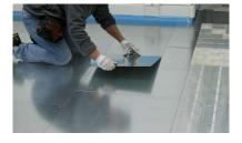
Steel sheet Limited thickness (2 mm) High conductivity Quick installation Relevant costs
